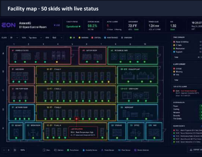
Facility map · 50 skids with live status 10x5 grid, zone colors, status dots, hover details
